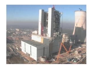
New 858 MW lignite-based, post-combustion capture, 2015, 1/3 CCS
